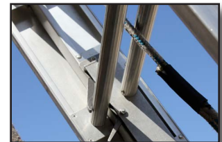
Figure 19-6 Lock position with the fly facing away from the building
