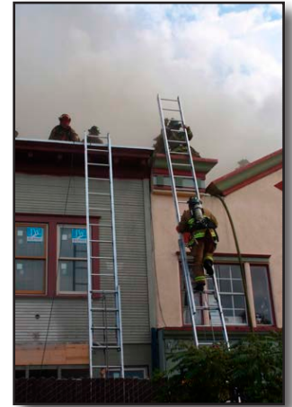
Figure 19-2 The ladder on the left is too short for this roof
