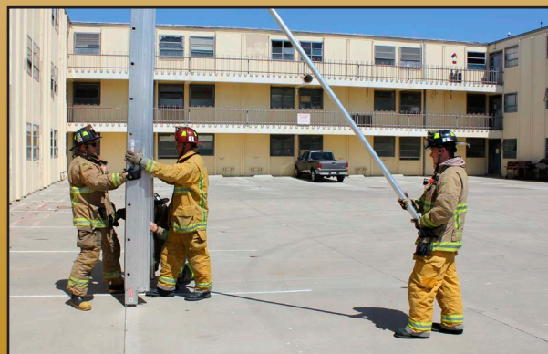
Walk the "pike" out to a 45 degree angle, one "pike" at a time
